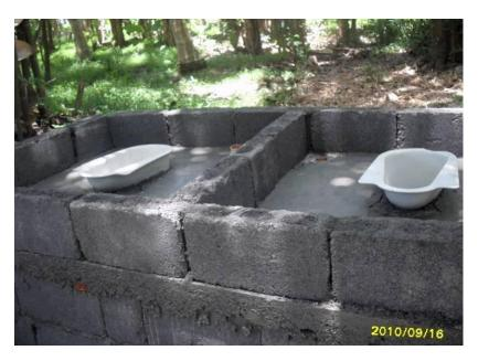
For low use situations the top of a pit is covered with a slab containing the water seal pan, vent pipe, and clean out pipe. The top of the pit can be lined to prevent the hole from collapsing but must be built to promote the leaching of water. A leach pipe can be installed similar to the photo above.
